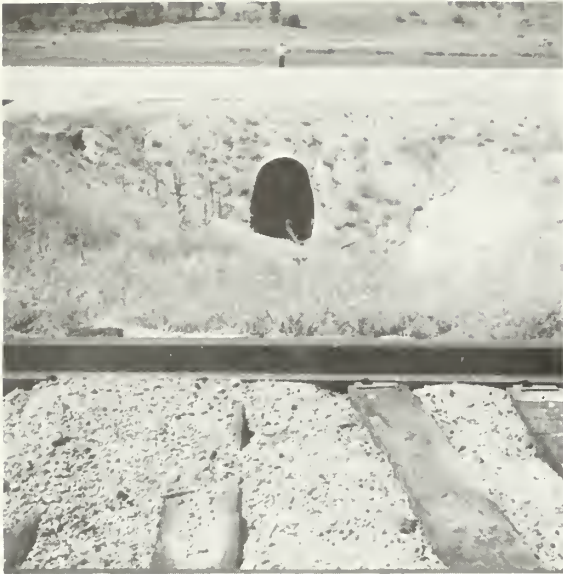
Looking westerly from railroad right-of-way; showing EAST ENTRANCE
